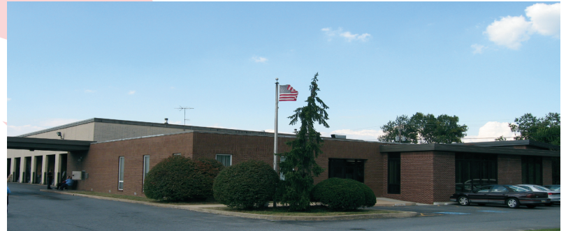
Former Operations Center
