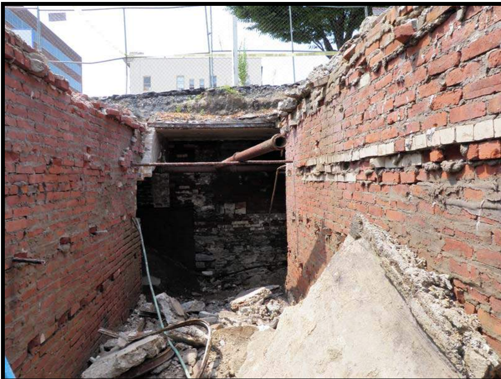
Figure 5.52 View looking west, showing probable gas line pipes for lighting in south wall of pedestrian tunnel.
