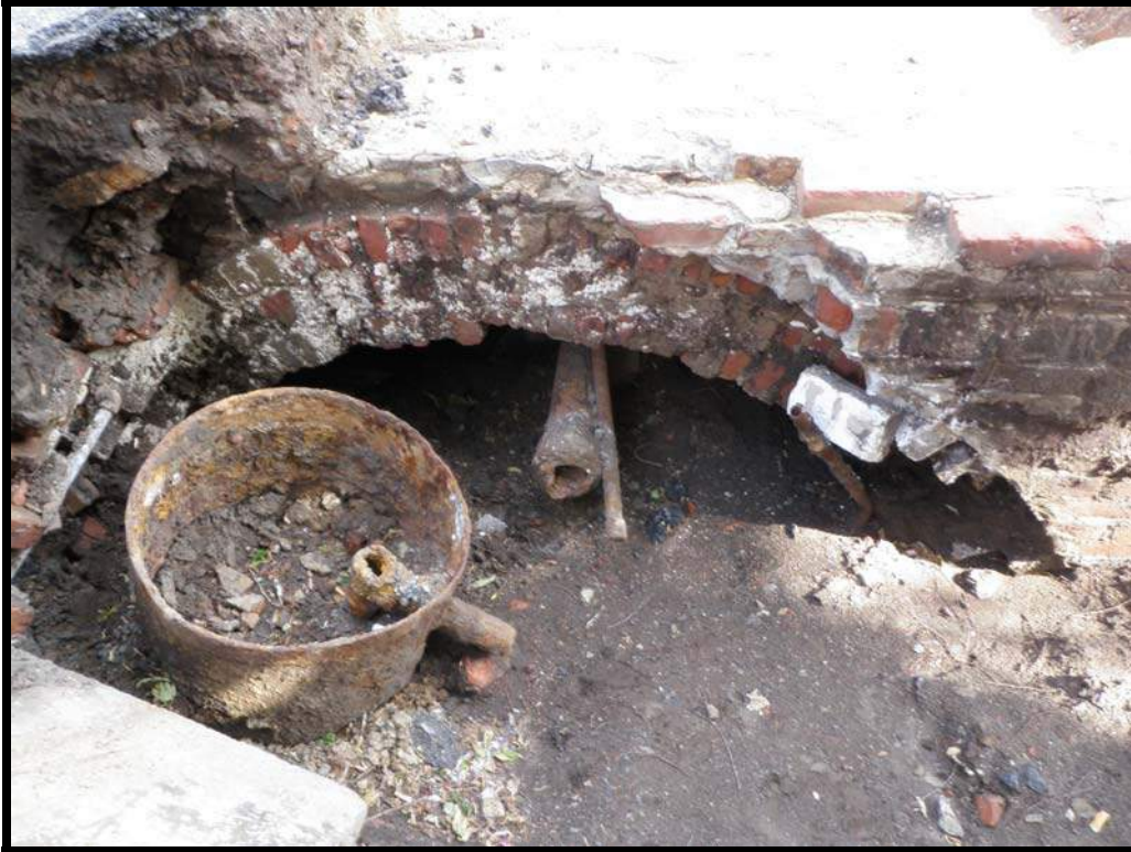
Figure 5.7 View facing north, showing the south pedestrian tunnel entranceway along Queen Street.
