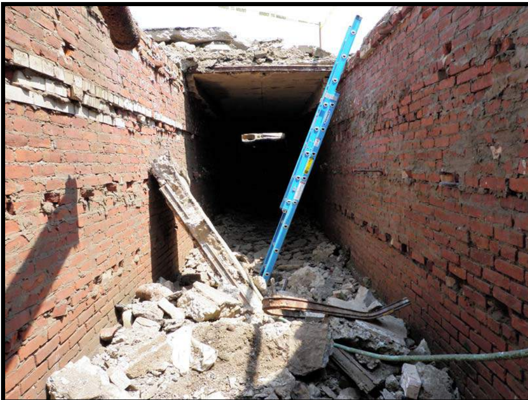
Figure 5.47 View looking west, showing the tunnel interior and floor accumulation.
