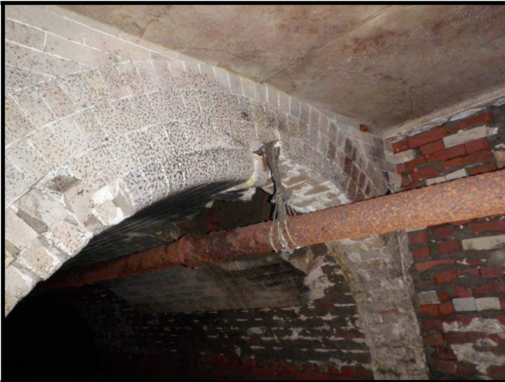
Figure 5.6 View facing southwest, showing the north vaulted pedestrian tunnel entranceway along Queen Street.
