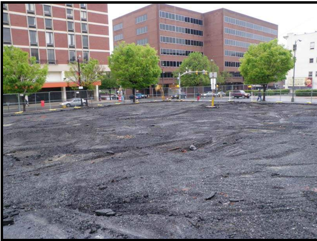
Figure 5.2 View facing southwest, showing the project site after asphalt removal.
