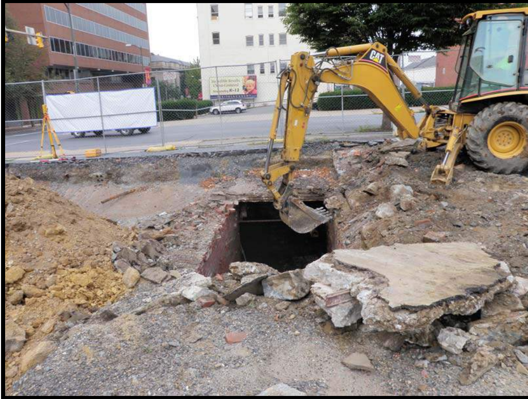
Figure 5.46 View looking west, showing machine removal of passenger tunnel roof.
