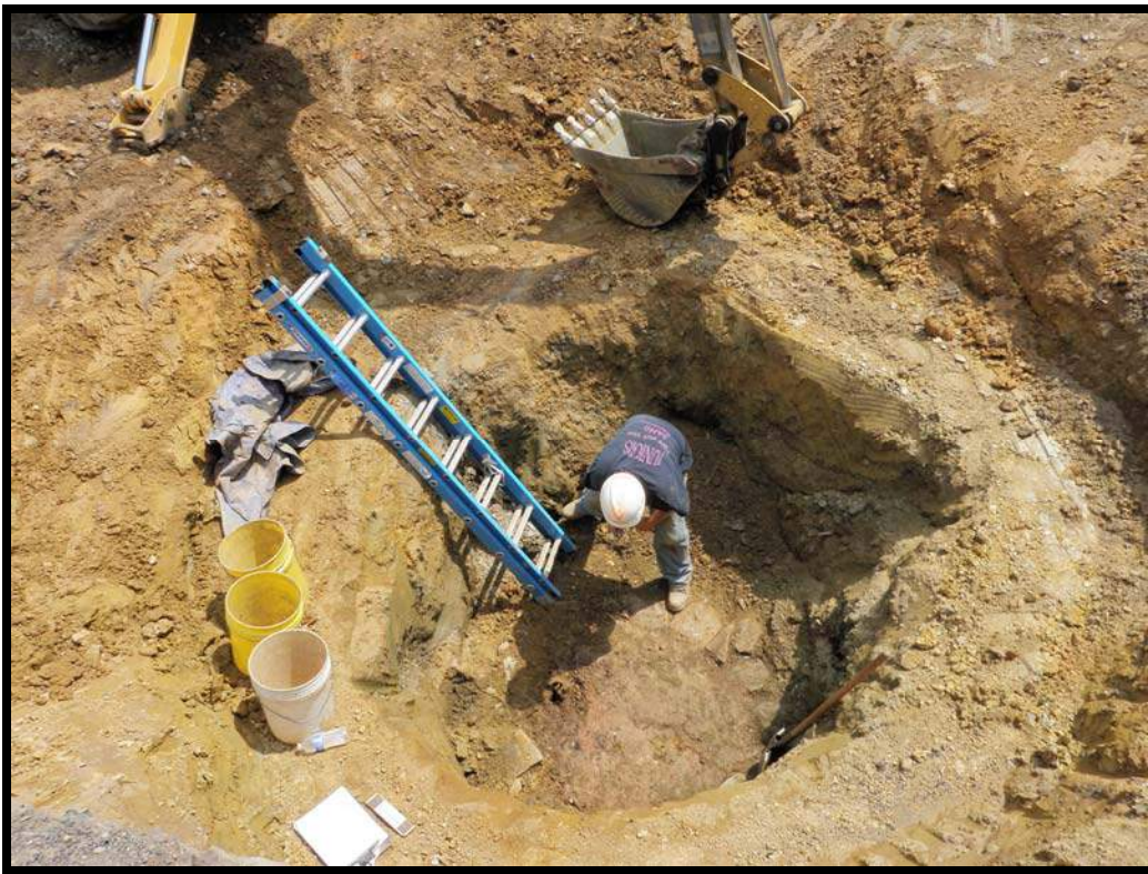
Figure 5.44 View showing benched area and well shaft during excavation.
