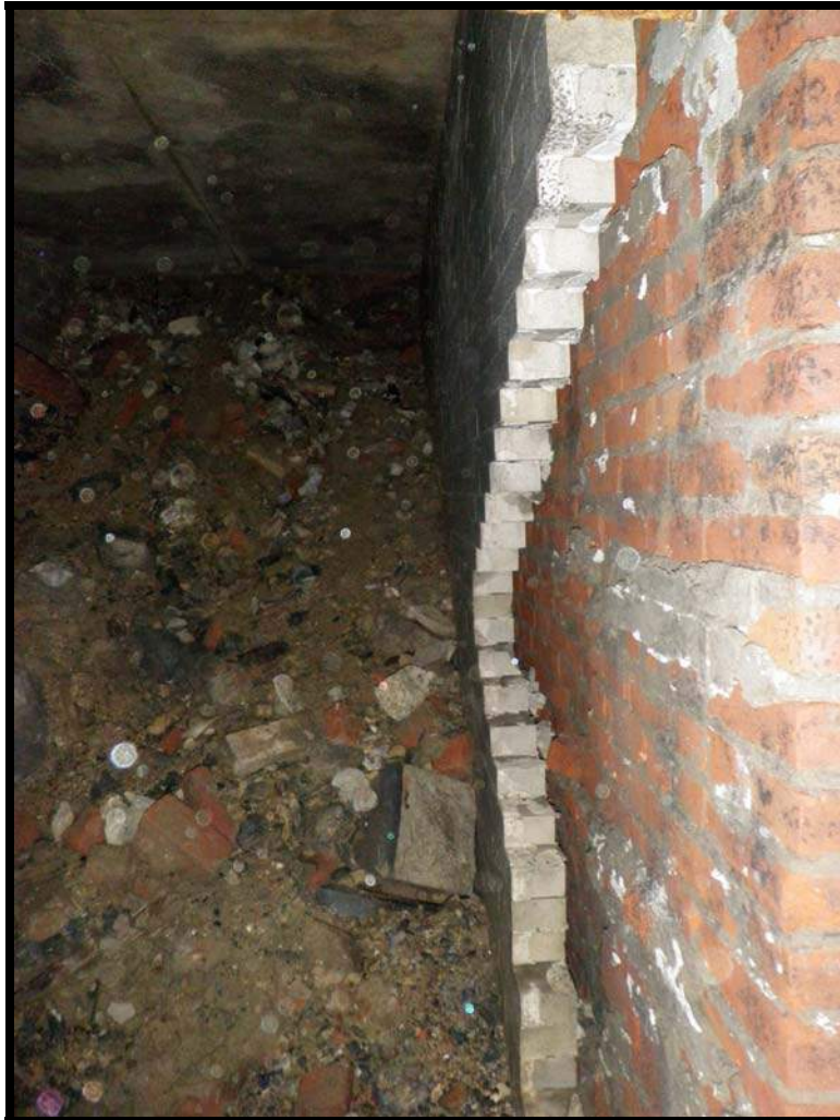
Figure 5.11 View facing north, showing decorative brick facing along the brick pedestrian tunnel wall.
