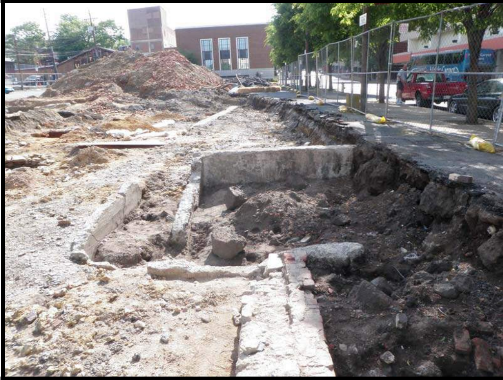
Figure 5.5 View facing east, showing the south stairwell foundation of the former train shed.
