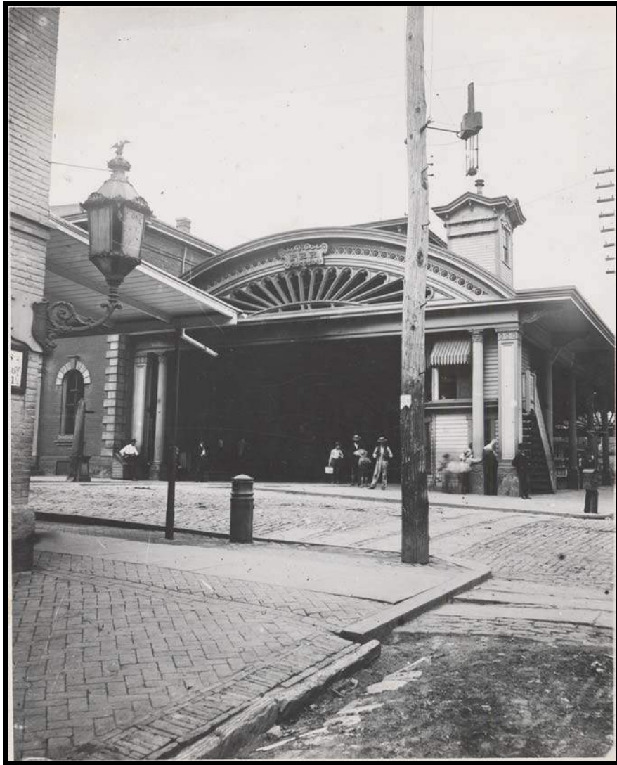
Figure 3.13 P.R.R. Lancaster Station, 1889. View looking east at the intersection of N. Queen and E. Chestnut Street. The building containing the waiting room and baggage areas is visible to the left of the train depot.
