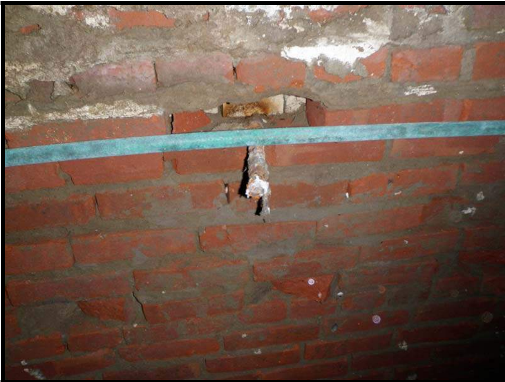
Figure 5.8 View showing a probable attachment point for a light fixture.
