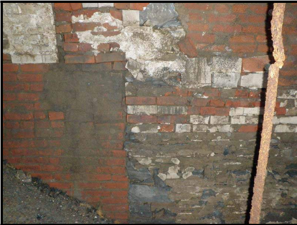
Figure 5.10 View facing west, showing the probable west wall foundation of the 1848 Lancaster City Exchange Hotel.
