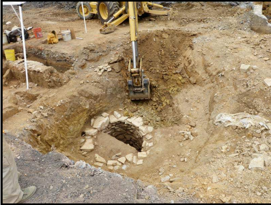
Figure 5.40 View showing mechanical excavation of Feature 2 well shaft.
