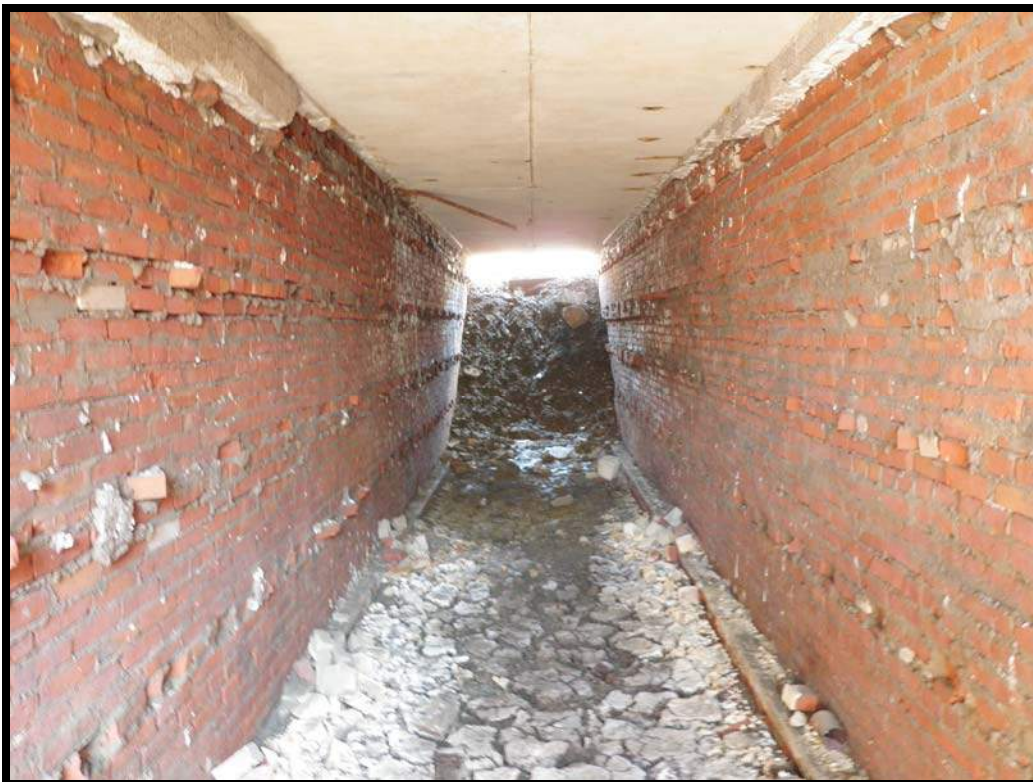
Figure 5.50 View looking east, showing east-west pedestrian tunnel in the direction of the stone stairwell.
