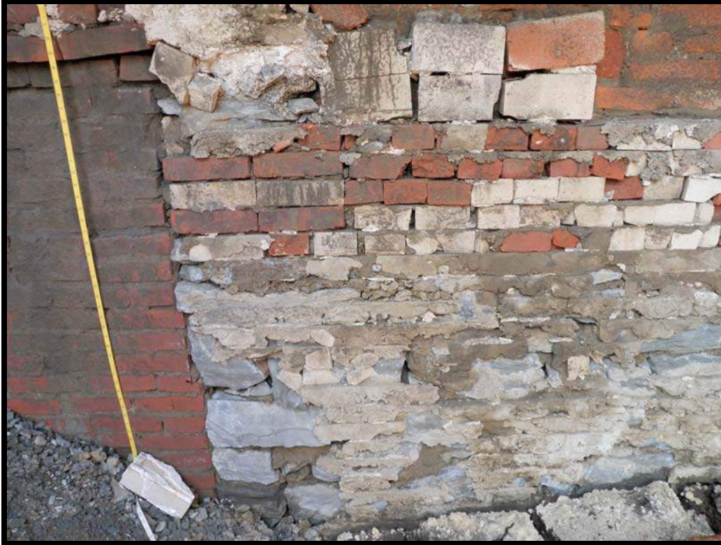
Figure 5.49 View looking west, showing possible remnant stone foundation wall of the Lancaster City Exchange Building.
