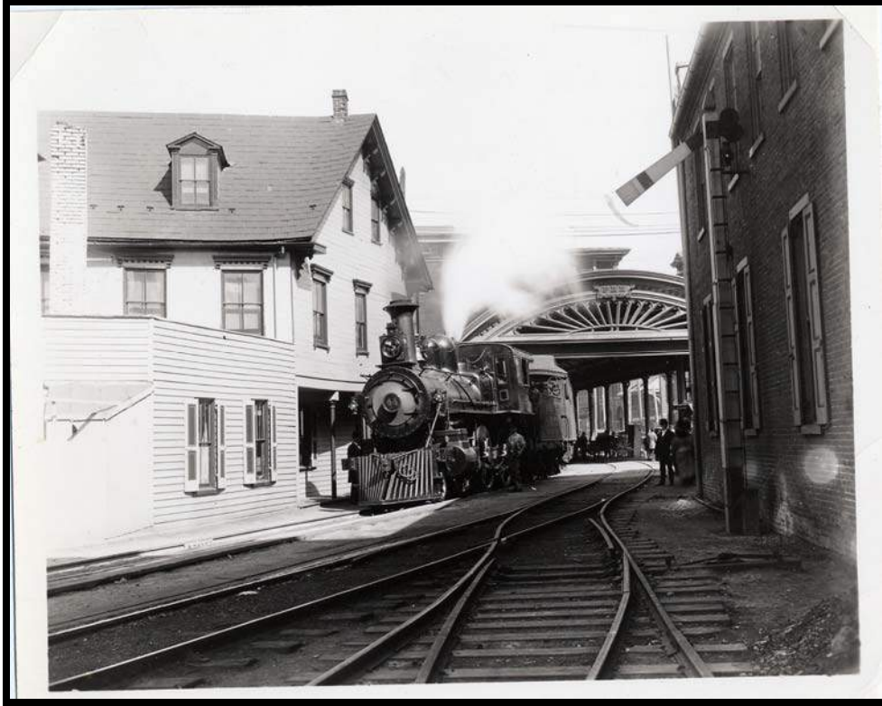
Figure 3.14 P.R.R. Lancaster Station, 1899. View looking east from the opposite side of Queen Street. The P.R.R. station/depot is visible in the background.
