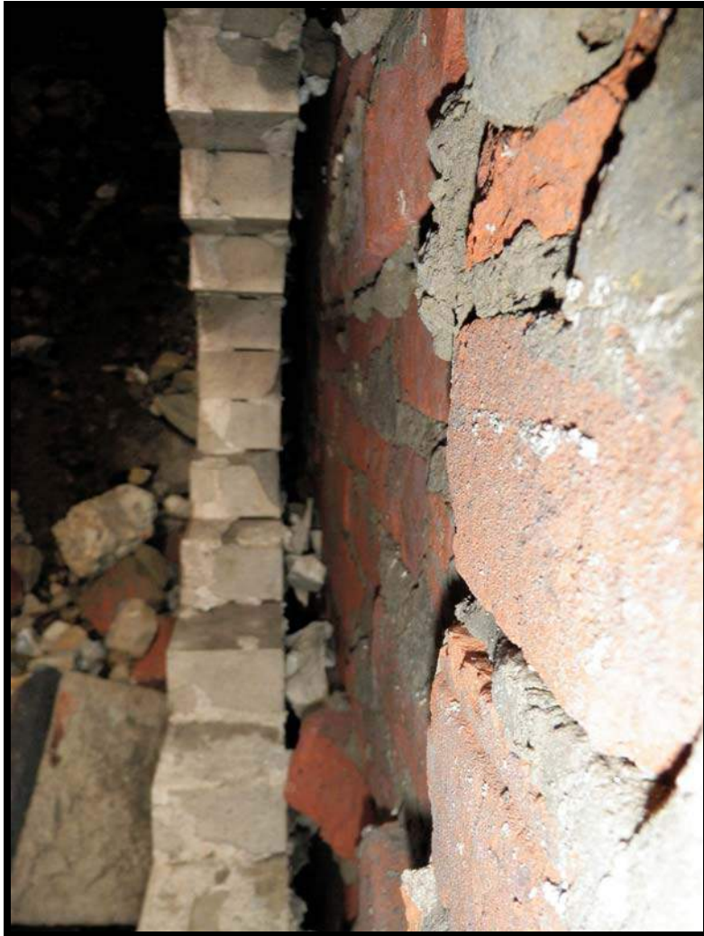
Figure 5.48 View showing a section of surviving white brick facing along passenger tunnel interior wall.
