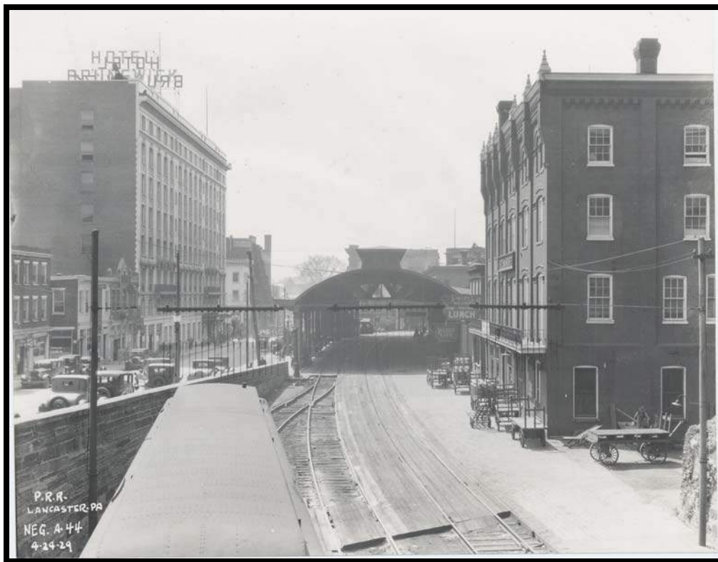
Figure 3.18 P.R.R. Lancaster Station, 1929. View looking west from Duke Street Bridge.
